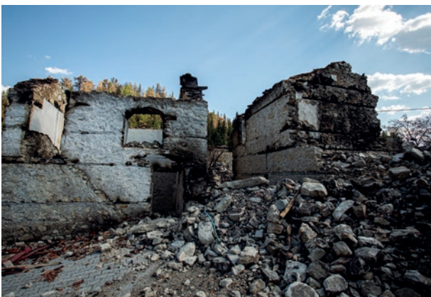
Wildfires in Antalya: a burnt building in Sevinçköy, Turkey.
